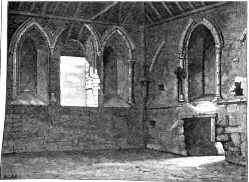
Internal View of the West End of Hardham Priory Chapel.
